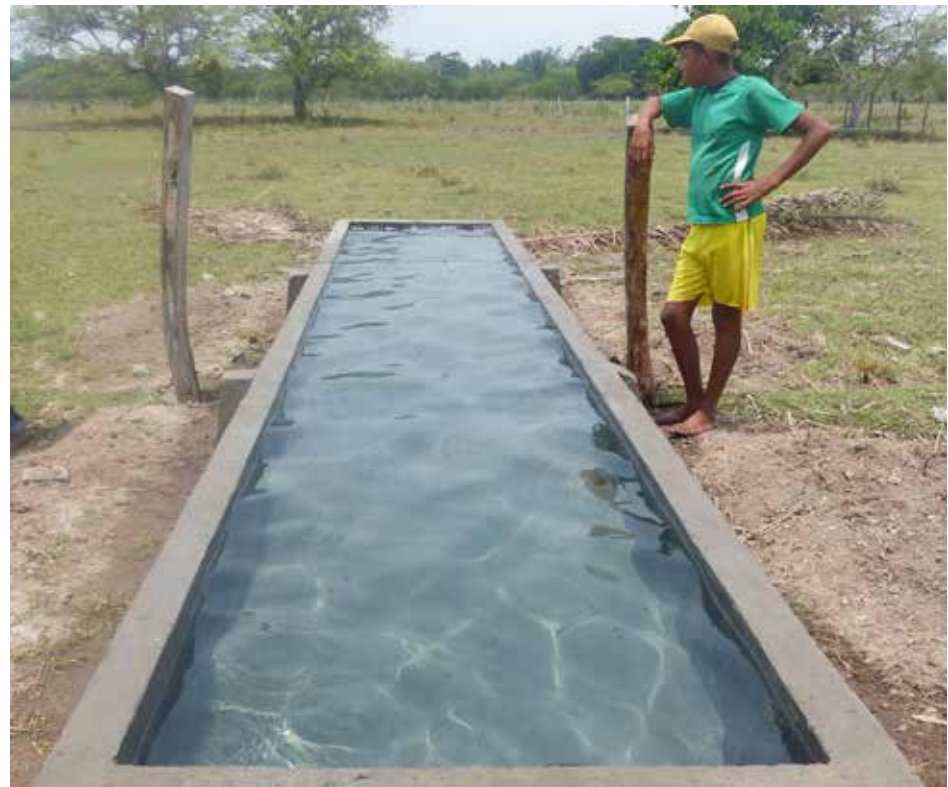
The newly built livestock watering system, built to prevent habitat degradation by livestock drinking from a stream inhabited by the Dahl’s Toad-headed Turtle. PHOTO CREDIT: RUBEN PALACIOS
