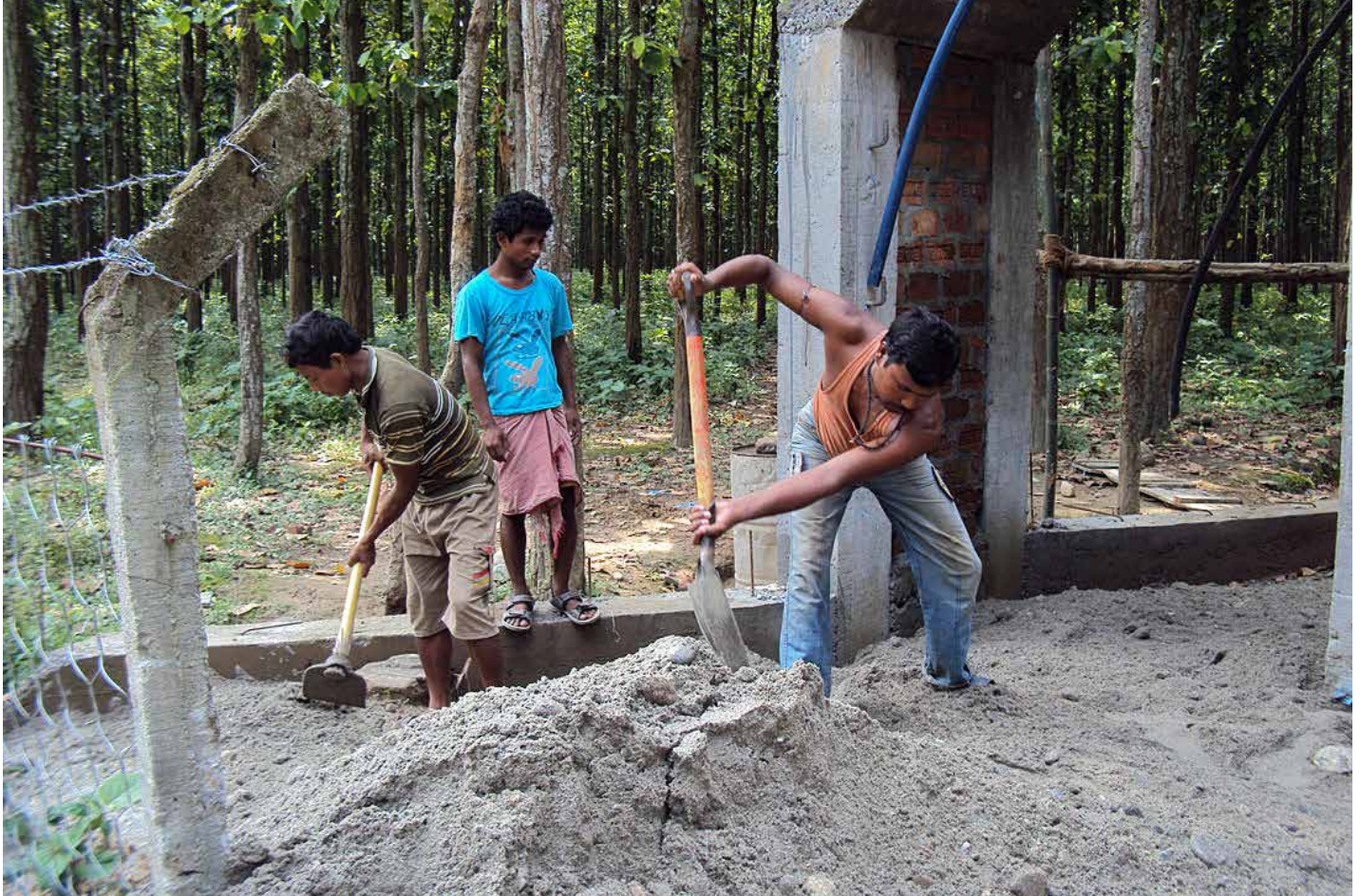
Construction is underway on a new turtle conservation center in Nepal. PHOTO CREDIT: ARCO NEPAL
