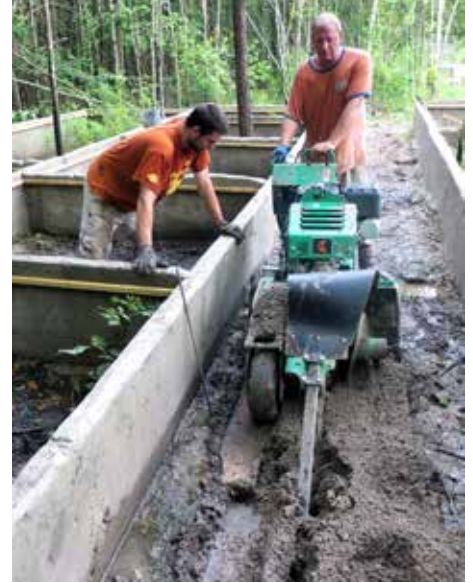
Jeff McKenzie and Luke Wyrwich are having a hard time using this Ditch Witch in muddy terrain, Construction progress has been hampered due to abnormally wet weather leading to frustrations. PHOTO CREDIT: RICK HUDSON
