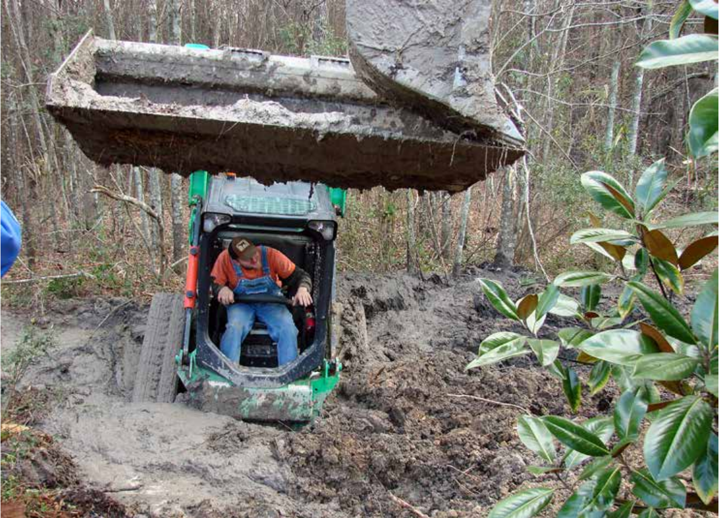
Abnormally high precipitation this year have created abysmal construction conditions. PHOTO CREDIT: CRIS HAGEN
