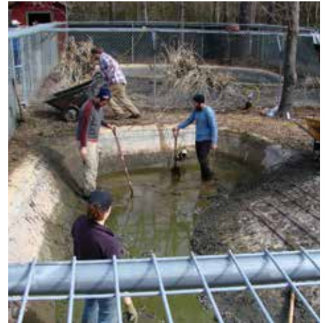
More than 20 tons of gravel were removed from former crocodile pools by dedicated volunteers. PHOTO CREDIT: CRIS HAGEN
