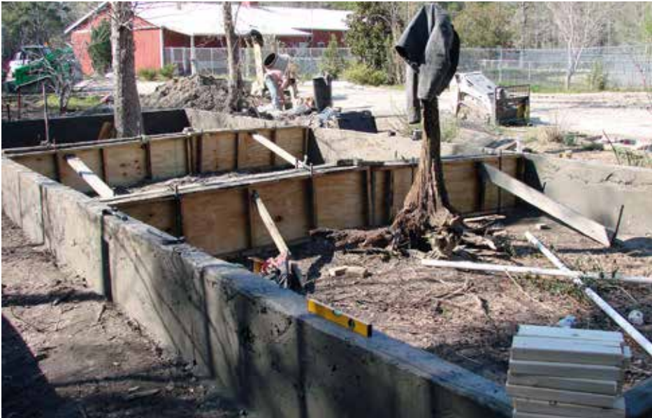
The walls of the Forest Complex being formed and poured during one of the few sunny days during the project. PHOTO CREDIT: CRIS HAGEN
