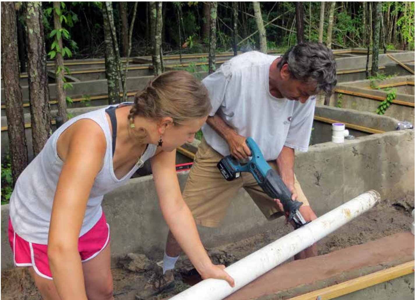
Jay Allen and Theresa Stratmann cutting PVC pipe for the drains to the Forest Complex PHOTO CREDIT: RICK HUDSON
